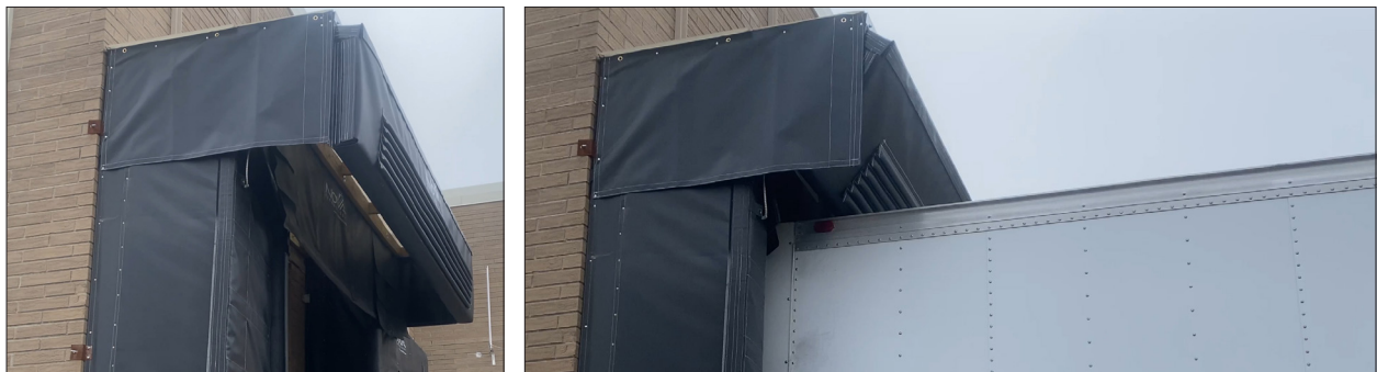
Multi-layer, foam-filled water defense system pivots with trailers as they approach the dock
