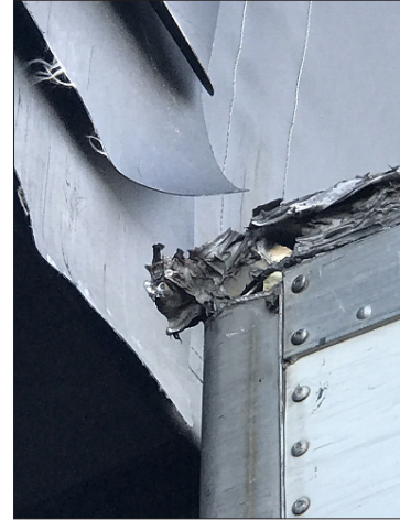
Trailer damage and irregularities create gaps where water can enter the dock
